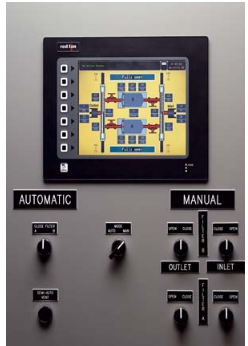
Control systems for MAAG's duplex filter
